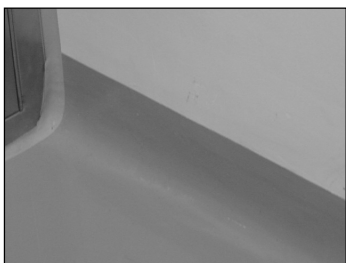
High density, smooth plaster, waterproofed by painting acrylic / high polymer enamel
